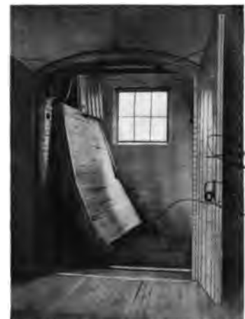
Fig. 3. Wrecked Elevator Car.
